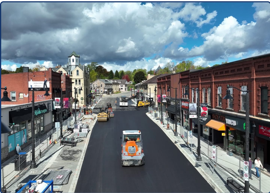
Fresh pavement on the Downtown Dig. Drone photo shared on Facebook.
