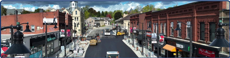
Fresh pavement on the Downtown Dig. Drone photo shared on Facebook.
